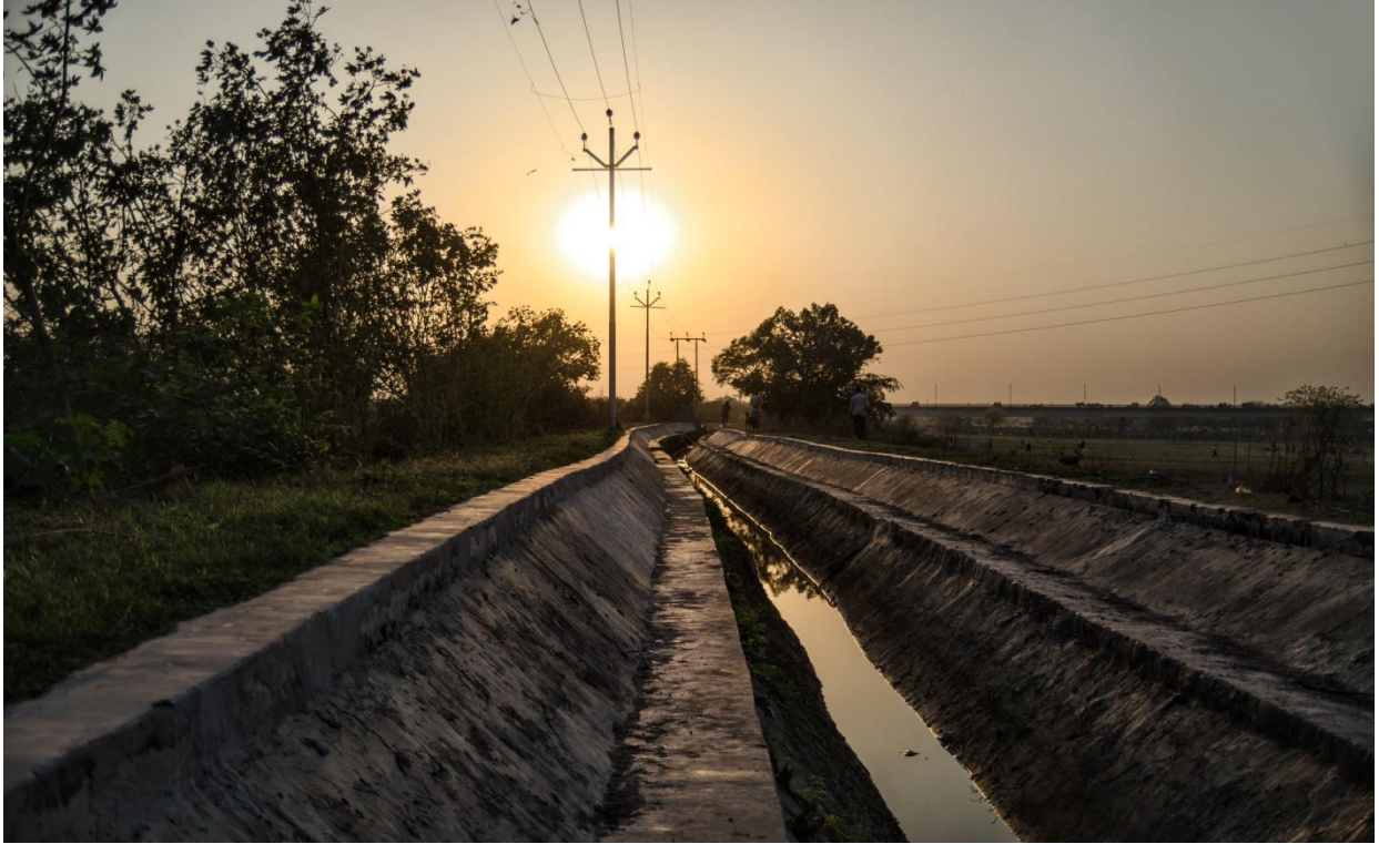
Figure 25: Water Channels built to transfer STP water to Rose farms
